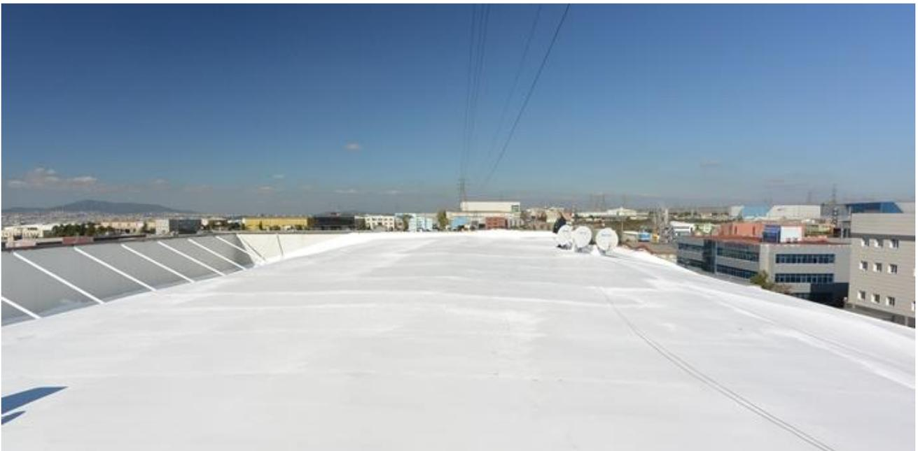
**COOL-R** was designed to achieve the **highest Solar Reflectance Index (SRI)**. The SRI is a function of two key parameters: **reflectivity, which is a measure of the ability to reflect solar radiation, and emissivity – the ability to release the absorbed heat.** Thanks to its unique technology, the innovative **COOL-R** coating has an very **high SRI of 107**. It is this value that demonstrates an efficiency that has been unattainable by the solutions available in the market to date.
